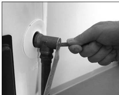
Figure 38 - T&P Relief Valve
