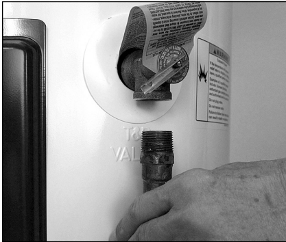
Figure 11 - Removing the T&P Relief Valve discharge pipe.
