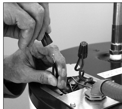
Figure 19 - Connecting the electrical wires.
