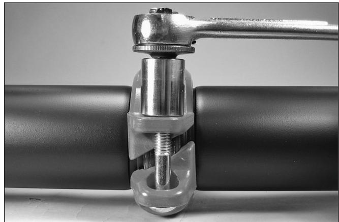
**5. ASSEMBLE JOINT:** Assemble the joint by inserting the grooved end of a pipe/mating component into each opening of the coupling. The ends of the grooved pipe/mating components must be inserted into the coupling until contact with the center leg of the gasket occurs. A visual check is required to ensure the coupling keys align with the grooves in the pipe/mating components. **NOTE:** The coupling may be rotated to ensure the gasket is seated properly.
