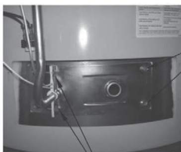
1/4" HEX DRIVE SCREWS AT FLANGE AREA OF INNER DOOR
