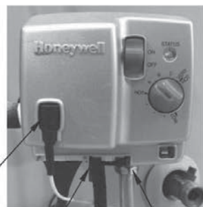
PILOT TUBING NUT FEEDLINE NUT
