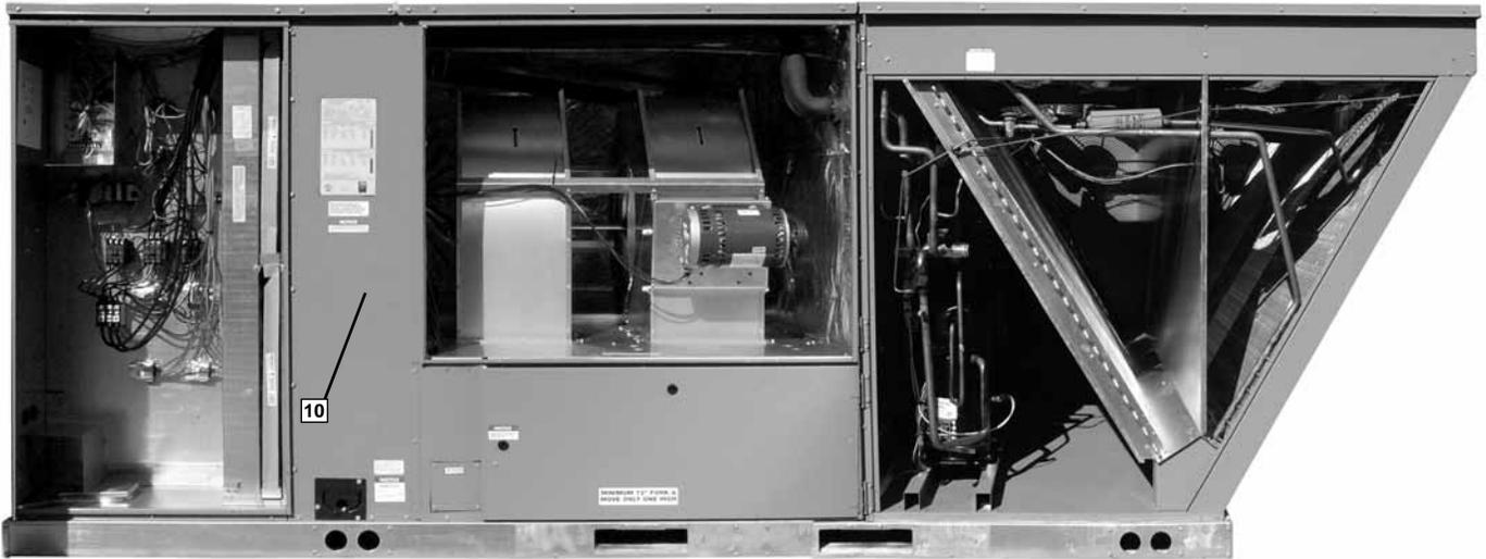
A control box component location legend sticker (11) is located on the left interior surface of the control section to match the components to the wiring diagram for ease of trouble shooting. Wiring is numbered on each end of the termination and color-coded to match the wiring diagram. The control transformer has a low voltage circuit breaker that trips if a low voltage electrical short occurs. There is a blower contactor and contactor for each compressor.
