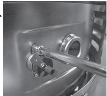
Step 6. Reconnect wire leads from combination thermostat/gas valve to resettable thermal switch.
