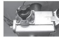
For White Rodgers mechanical control, depress knob slightly and rotate clockwise to the "OFF" position.
