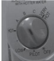
For White Rodgers mechanical control, depress knob slightly and rotate clockwise to the "OFF" position.
