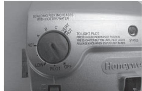
Rotate knob counter-clockwise to the "OFF" position
