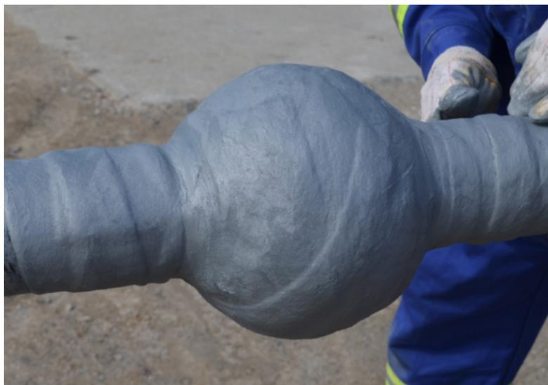
Use of Fill-Pro™ PM-GP profiling mastic creates a uniform profile for the application of Trenton Wax-Tape® anticorrosion wrap.
