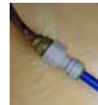
standard cold side connection from the faucet to Max Flow using included fitting (see above) and inserted blue tubing 1
