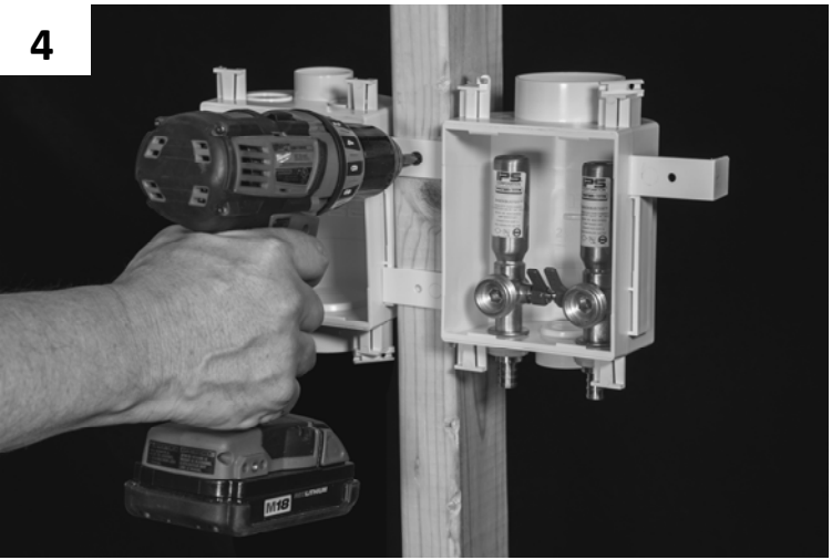
4 Straddle the stud and secure the box thru the integrated flanges' screw hole. For additional securement, insert nails through nail slots.
