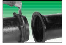
Clean the socket and the plain end. Lubrication is recommended for proper assembly of all mechanical joints. Lubrication and additional cleaning should be provided by brushing both the gasket and plain end with soapy water or pipe lubricant just prior to slipping the gasket onto the plain end for joint assembly. Place the gland on the plain end with the lip extension toward the plain end followed by the gasket with the narrow edge of the gasket toward the plain end.
