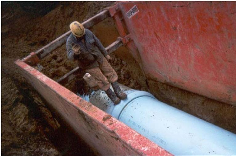
Photo 10 (Large Diameter Joint Assembly)
