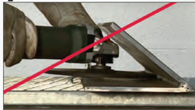
Typical solution violates safety standards
