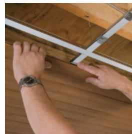
Position planks; slide and secure clips
