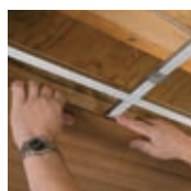
Position planks; slide and secure clips
