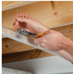
2 Suspend main beams with hanging hardware
