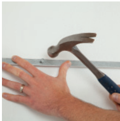
1 Install wall molding
