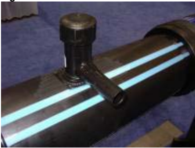
Figure 11: Saddle Fusion of PE Water Service Line to Main
