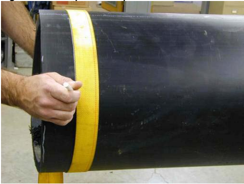
Figure 50: Cut Pipe Ends Square
