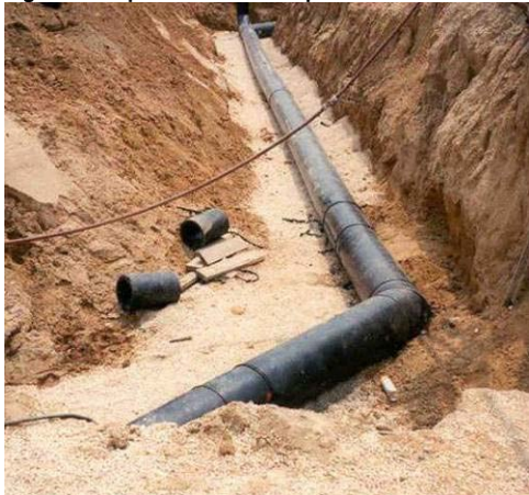
Figure 21: Pipe Placement in Open Trench
