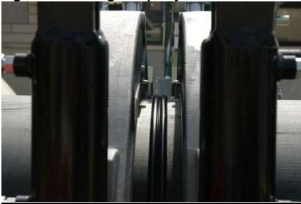
Figure 36: Joining of Pipe by Butt Fusion
