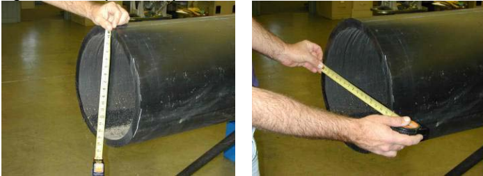
Figure 52: Cut Pipe Ends Square
