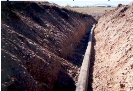
Figure 23: Trench Wall Sloped for Safety
