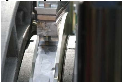
Figure 35: Melting of Pipe for Fusion
