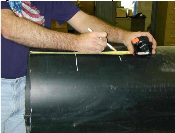
Figure 51: Mark Insertion Depth on the Pipe
