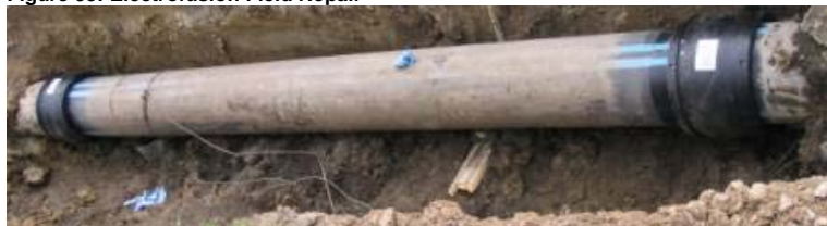
Figure 93: Electrofusion Field Repair
