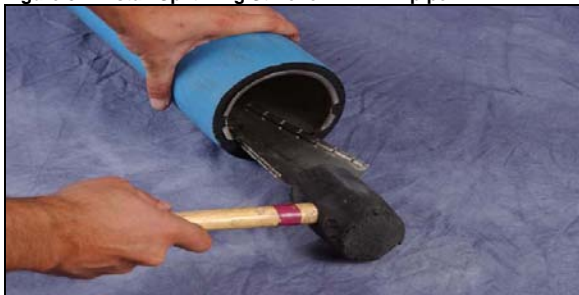
Figure 87: Install Split Ring Stiffener in HDPE pipe
