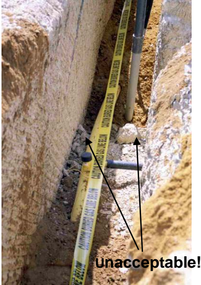
Fig. 25: Avoid Rock Impingement when Placing Embedment
