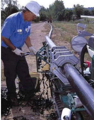
Figure 31: Butt Fusion of Water Pipe
