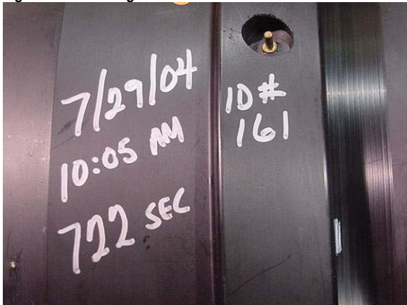
Figure 58: Recording the Electrofusion Information
