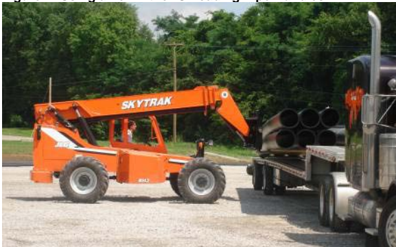
Figure 4: Using a Forklift for Unloading Pipe Bundles
