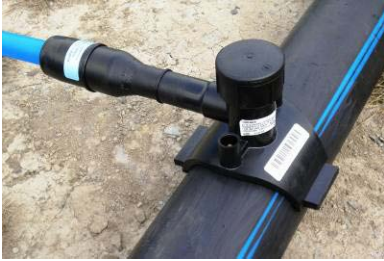
Figure 12: Saddle Electrofusion of PE Water Service Line to Main
