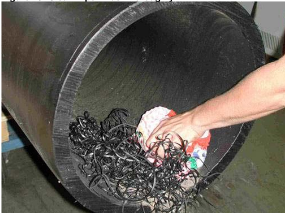
Figure 49: Clean Pipe Ends Thoroughly
