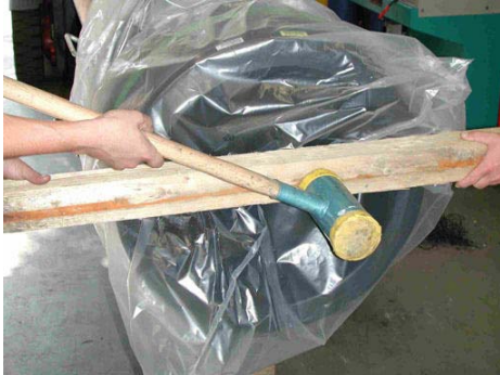
Figure 56: Installing Coupler on Pipe
