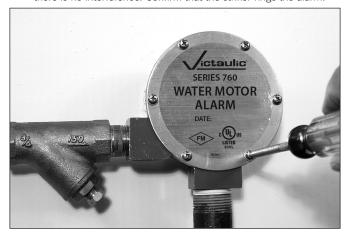
18. Install the cover plate onto the alarm motor housing. Install and tighten the six screws to secure the cover plate to the alarm motor housing.
