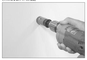
1. Drill a 1¼-inch/32-mm hole in the appropriate location for the connecting nipple. In addition, drill a 1½-inch/41-mm hole in the appropriate location for the 1-inch/33.7-mm diameter drain nipple.
