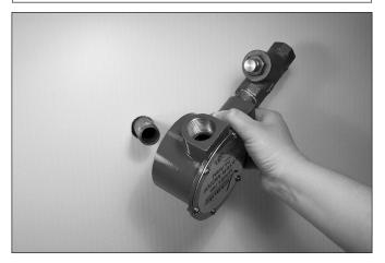
From the interior of the building, hand-tighten the alarm motor housing onto the end of the connecting nipple.
