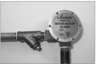
**14.** Install the 1-inch/33.7-mm diameter drain piping from the alarm motor housing's outlet to the drain location. **NOTE:** The drain must discharge through an open fitting.
