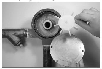
**15.** Remove the six screws from the cover plate. Remove the cover plate and impeller. Verify that the factory-installed, non-hardening pliable sealant is intact within the groove in the alarm motor housing. If the sealant is not in good condition, remove all material and re-apply sealant/caulk into the groove, as needed.
