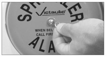
12. Install the flat washer and lock washer onto the threaded stud of the bracket.
