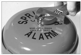
**8.** Tighten the shell securely with the supplied fastener.
