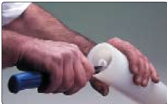
Figure 3: Chamfer the Tubing
