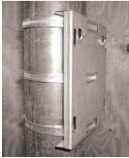
Ensure that the hooks are on the top and that all three straps are fastened tight against the riser (no slack).
