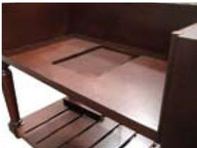
3. The most common installation design is undermounted below the solid surface. Using the sink to be installed, measure where to install the support frame. (Fig.1) Shimming may be necessary to move the sink up to the solid surface or to make the sink drain properly. A reveal of 1 to 2 inches is common. (Fig. 2)
