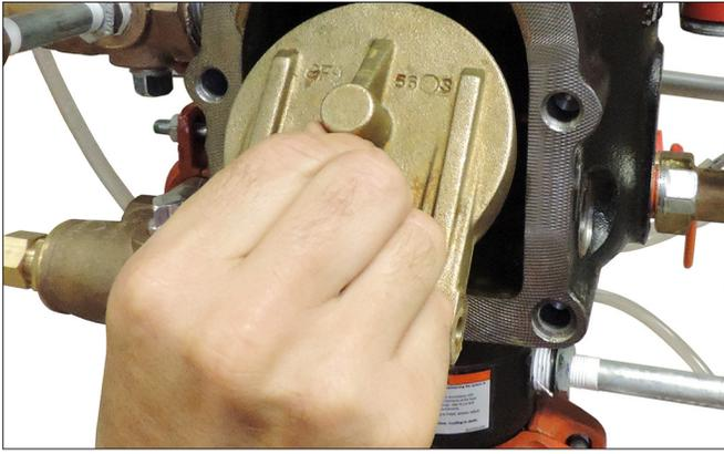
4. Remove the clapper assembly from the valve body seat ring. Clean the valve body seat ring.
