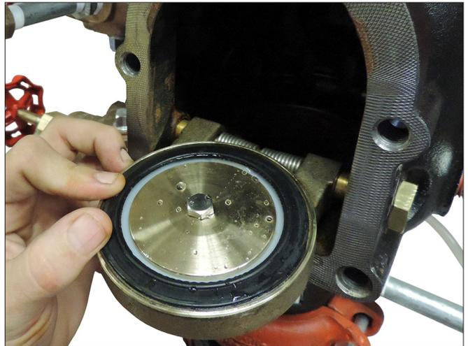
14. Rotate the clapper out of the valve body. Inspect the clapper seal and seal-retaining ring. Wipe away any contaminants, dirt, and mineral deposits. Clean out any holes that are plugged in the valve-body seat ring. **DO NOT USE SOLVENTS OR ABRASIVES.**
