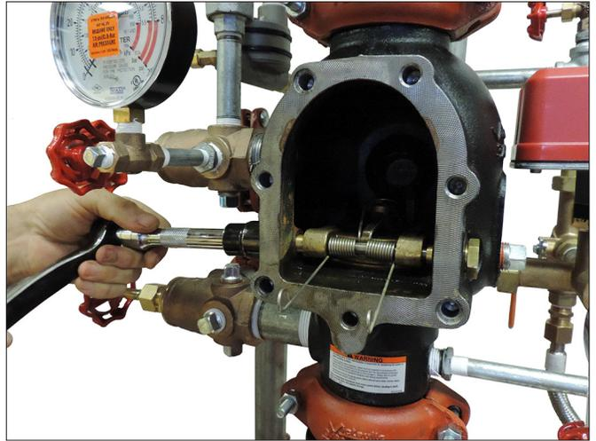
9. Ensure that a clapper shaft bushing o-ring is installed on each clapper shaft bushing.
