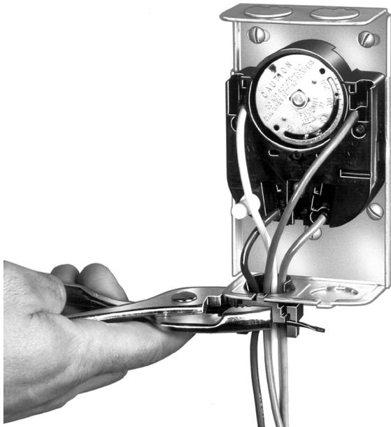
Fig. 8. CLOSING THE STRAIN RELIEF BUSHING.
