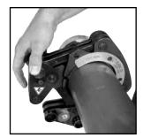
**6.** Select the correct size pressing chain. Pull the pin on the chain which allows the segments to open. Position the chain on the raised bead and wrap the chain around the fitting with the "pipe side" designation facing the tube. When the chain is fully wrapped around the fitting, reinsert the pin to secure the chain on the assembled joint. Visually inspect the mark made in Step 5 to ensure the tube remained in position.
