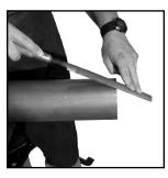
3. Deburr the tube outside diameter using a half-round file to prevent damage to the EPDM seal. Clean the tube end of all contamination, oils, shavings and oxidization. A smooth transition chamfer is recommended to ease tube insertion past the seal.
