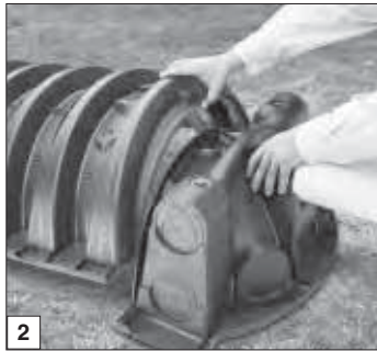
2 Place first chamber onto end cap.
