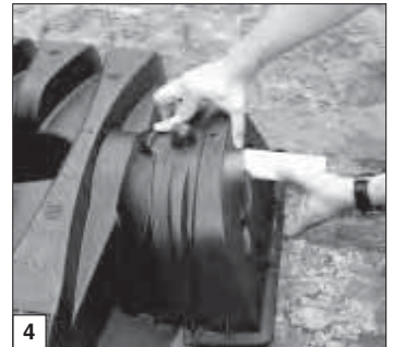
Place end cap over inlet end.
