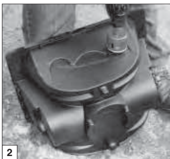
Drill pressure pipe hole.
