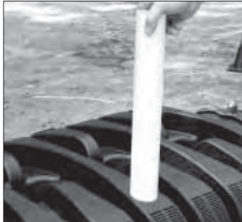
Chamber inspection port.
