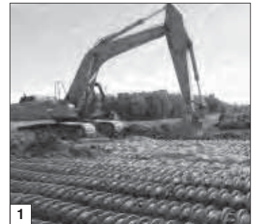
1 Ladle the fill.
