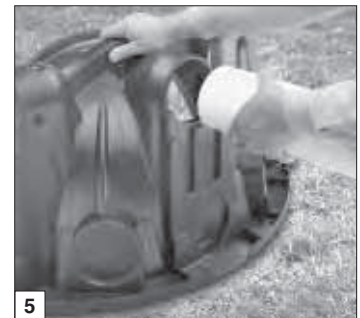
5 Insert inlet pipe.
