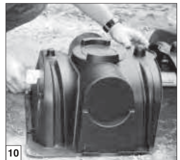
Lateral pipe through end cap.
