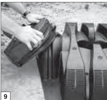
Place end cap outlet end.
