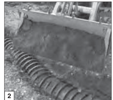
Backfill the soil.
