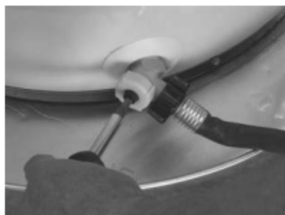
Figure 12 - Draining the old water heater.
