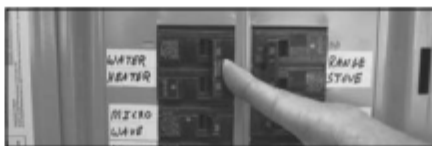
Figure 31 - Circuit Breaker
