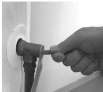
Figure 46 - T&P Relief Valve
