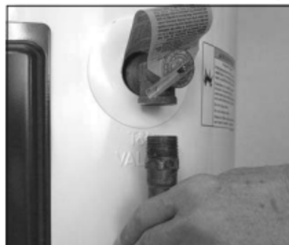
Figure 13 - Removing the T&P Relief Valve discharge pipe.
