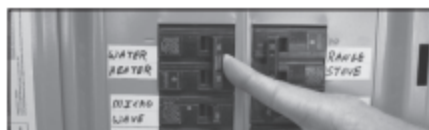
Figure 38 - Circuit Breaker
