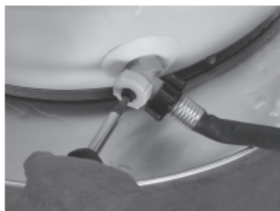
Figure 12 - Draining the old water heater.
