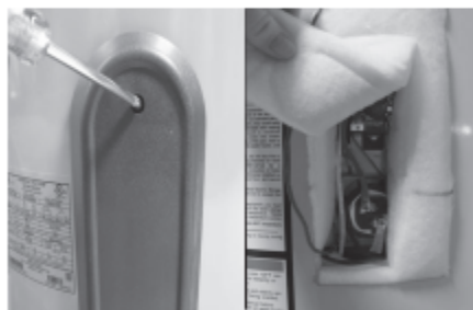
Figure 45 - Element Access Panel/ECO Compartment
