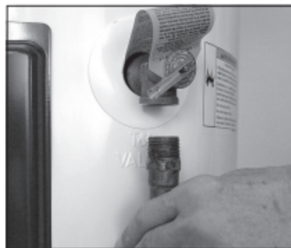
Figure 13 - Removing the T&P Relief Valve discharge pipe.
