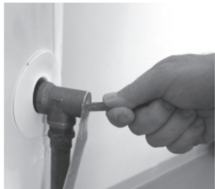
Figure 46 - T&P Relief Valve
