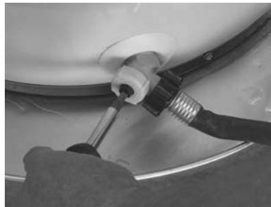
Figure 12 - Draining the old water heater.
