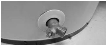
Figure 42 - Drain Valve
