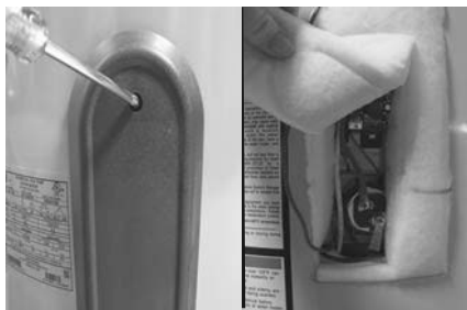
Figure 45 - Element Access Panel/ECO Compartment
