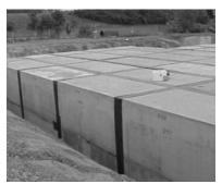
Membrane Waterproofing and Exterior Joint Wrap for Precast Concrete Joints
