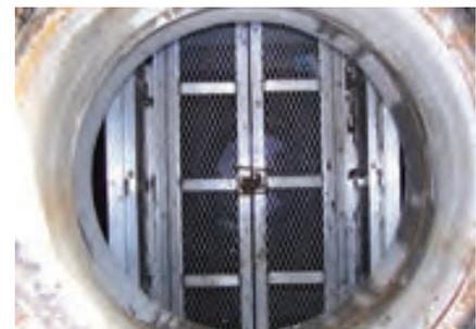
After cleaning sediment chambers, close and secure bottom screen doors to prevent debris loss.
