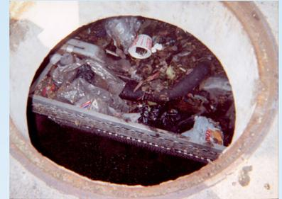
Standard Capacity Curb Inlet Basket™ installed under the manhole cover, full of trash and debris and ready for servicing.
