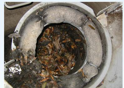
High Capacity Curb Inlet Basket™ full of debris and needs to be cleaned. The StormBoom™ is discolored indicating the need for necessary replacement.
