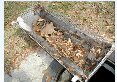
Standard Capacity Curb Inlet Basket™ removed from shelf inside inlet. The filtration basket holds dried debris ready to be disposed of and screen cleaned.
