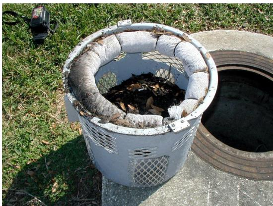
The shelf system allows for easy access to each Curb Inlet Basket™ for manual servicing.
