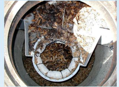
High Capacity Curb Inlet Basket™ after storm event containing dry foliage and debris ready for collection and disposal.
