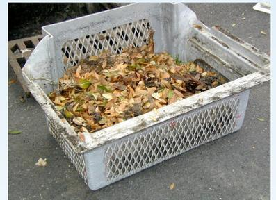
Grate Inlet Skimmer Box™ filtration basket removed by hand for manual disposal of debris and basket cleaning.
