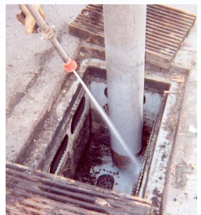
Grate Inlet Skimmer Box™ filtration basket being cleaned via vacuum truck hose and screens washed with spray wand.
