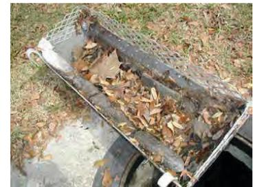
Standard Capacity Curb Inlet Basket removed from shelf inside inlet. The filtration basket holds dried debris ready for disposal.
