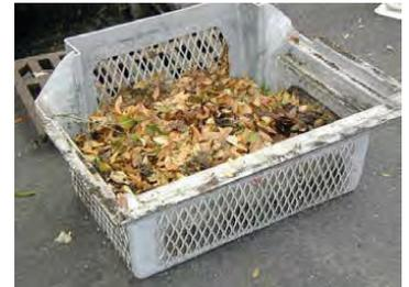
Grate Inlet Skimmer Box filtration basket removed by hand for manual disposal of debris and basket cleaning.
