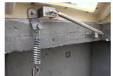
20 Attach cable to bracket
