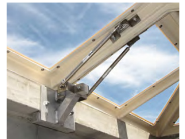
9 Attach center bracket
