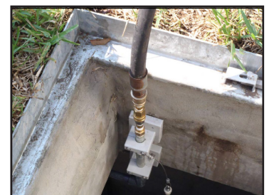
HydroSlide quick connector with vacuum truck water supply hose attached for sediment removal.
