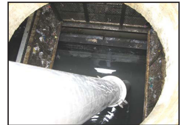
Open lower screen panels to remove sediments via vacuum truck.
