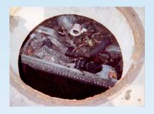
Standard Capacity Curb Inlet Basket™ installed under the manhole cover, full of trash and debris and ready for servicing.
