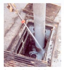
Grate Inlet Skimmer Box™ filtration basket being cleaned via vacuum truck hose and screens washed with spray wand.
