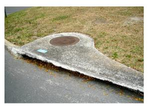
Curb inlet where servicing can only occur via access from the manhole.
