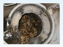
High Capacity Curb Inlet Basket™ full of debris and needs to be cleaned. The StormBoom™ is discolored indicating the need for necessary replacement.
