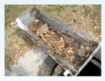
Standard Capacity Curb Inlet Basket™ removed from shelf inside inlet. The filtration basket holds dried debris ready to be disposed of and screen cleaned.
