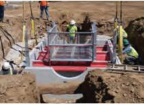
Fast set: pre-installed internal components (optional)
