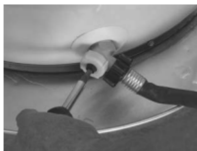
Figure 12 - Draining the old water heater.
