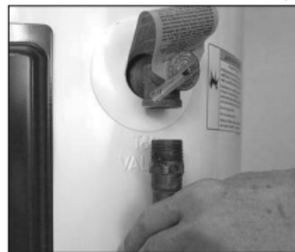
Figure 13 - Removing the T&P Relief Valve discharge pipe.
