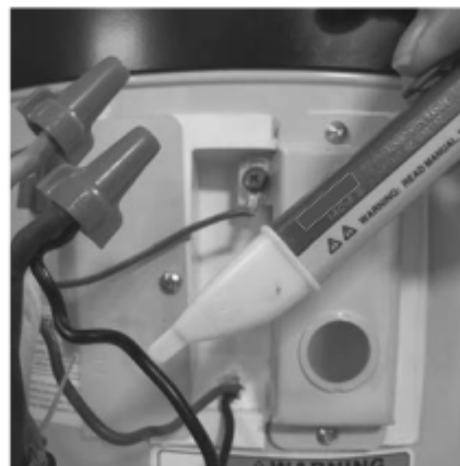
Figure 39 - Non-Contact Circuit Tester
