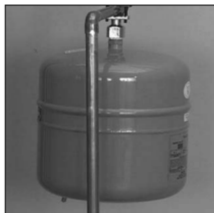
Figure 20 - The Thermal Expansion Tank should be pressurized with air, to match the home's incoming water pressure.
