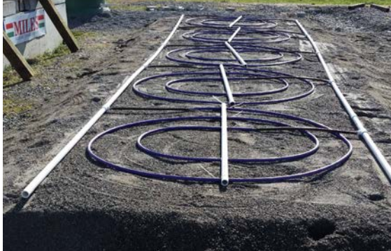
Manifolds and supply lines are 1" Sch 40 PVC
