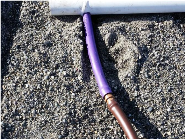
Blank tech liner and Bioline connection with internal coupling
