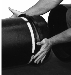
FIELD ASSEMBLY OF FLEX-RING
