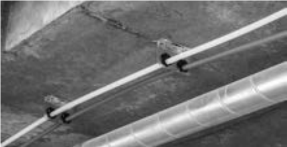
Figure 24: Supporting small-diameter coiled PEX
