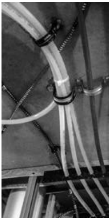
Figure 30: Proper bundling of Uponor PEX
