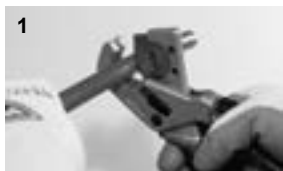
Figure 5: Square cut the pipe.
