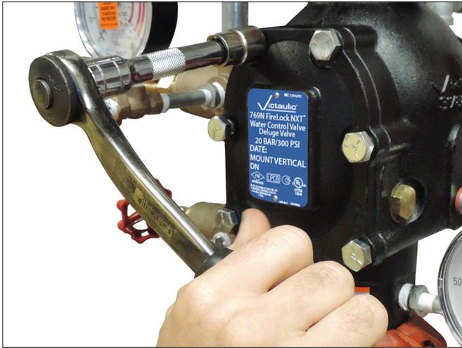
4. Align the cover plate/cover plate gasket to the valve. Verify that the clapper spring's arms are rotated to their installed position. Tighten all cover plate bolts into the cover plate/valve body.
