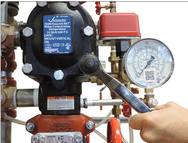
11. After all pressure is released from the system, loosen the cover plate bolts slowly. **NOTE:** DO NOT remove any cover plate bolts until all cover plate bolts are loosened.
