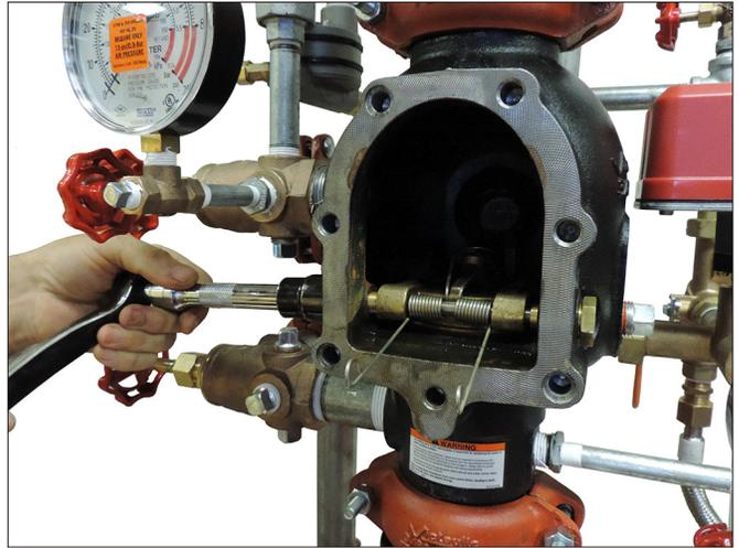
9. Verify that a clapper shaft bushing o-ring is installed on each clapper shaft bushing.
