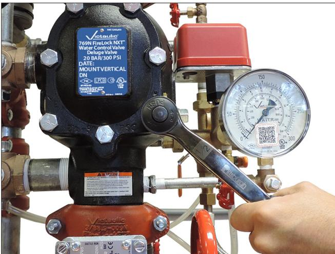
11. After all pressure is released from the system, loosen the cover plate bolts slowly. **NOTE:** DO NOT remove any cover plate bolts until all cover plate bolts are loosened.
