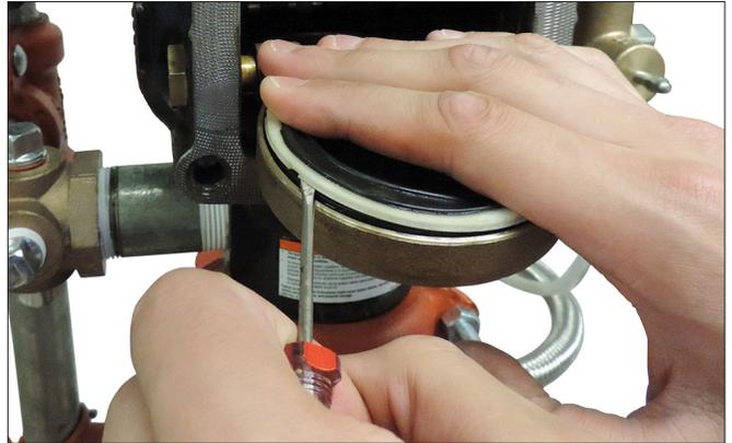
6. Pry the clapper seal, along with the seal ring, out of the clapper. Inspect the clapper seal. If the clapper seal is torn or worn, replace it with a new, Victaulic-supplied clapper seal. If replacing the clapper seal assembly with a new assembly, skip to step 7.
