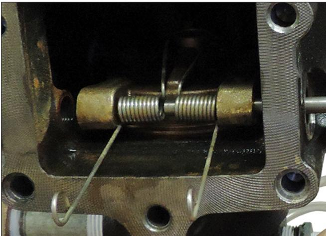
6. Insert the clapper shaft halfway into the valve body.
