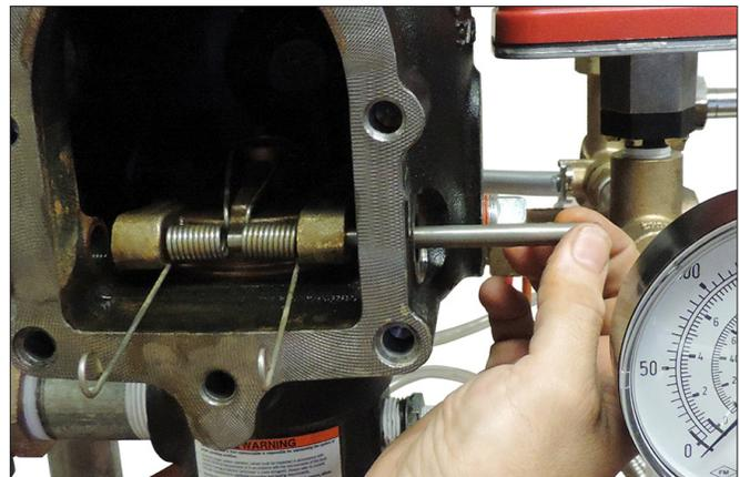
3. Remove the clapper shaft. **NOTE:** As the shaft is being removed, the clapper spring will drop out of position. Save the clapper spring for re-installation.
