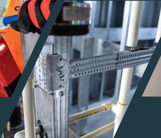
Secondary Pipe Supports
