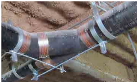
No-Hub Fitting Restraint
