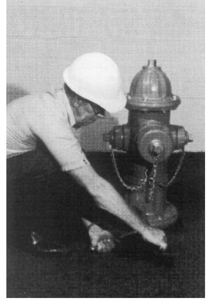
5. Tighten Safety Flange Bolts.
