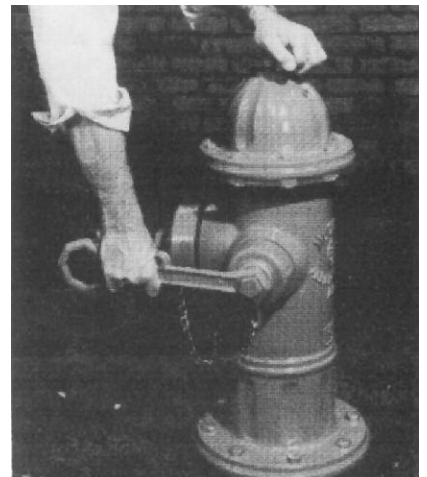
7. Replace and tighten Nozzle Cap.
