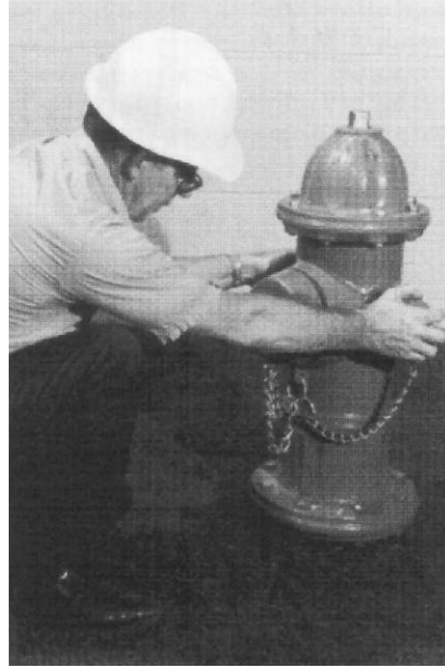
3. Rotate Upper Barrel section as desired.
