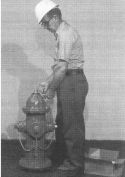
1. Remove Oil Filler Plug and check oil level. Oil should be level with Oil Filler Plug Hole.
