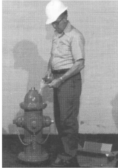
2. If oil is low, use a small funnel to add MUELLER Hydrant Lubricant
