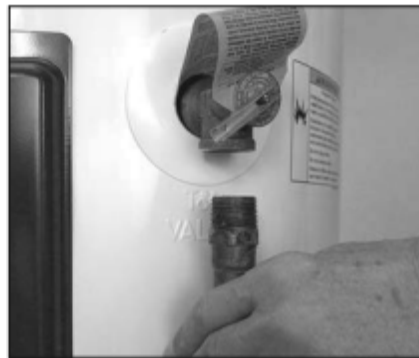
Figure 13 - Removing the T&P Relief Valve discharge pipe.
