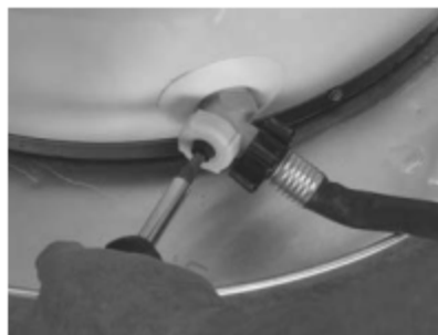
Figure 12 - Draining the old water heater.
