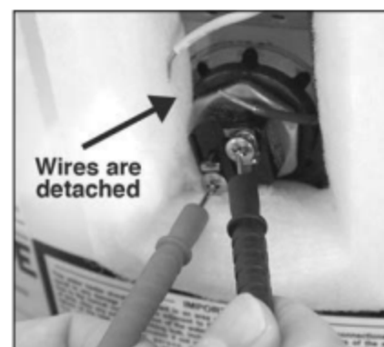
Figure 27 - Use a multi meter to check the resistance of the upper heating element.
