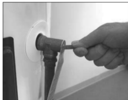
Figure 46 - T&P Relief Valve
