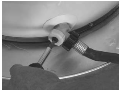
Figure 12 - Draining the old water heater.
