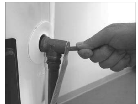
Figure 46 - T&P Relief Valve
