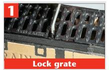
To close, place hook part of tool into 'V' and push towards rail.
