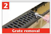
To remove grates, use wrench or socket set. Carefully store bolts for refitting of grates.
