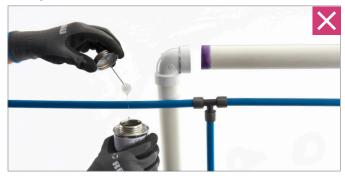
Ensure that the employed sealants, cleaning agents, building foams, insulation, protective tape, adhesive tape or thread sealant do not contain any components which cause stress cracking or corrosion, such as ammonia, ammonia-bearing, aromatic and oxygenated solvents (e.g., ketone and ether), chlorinated hydrocarbons or chloride ions which can leach.
