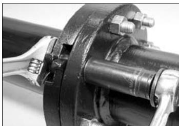
7. INSTALL REMAINING BOLTS/ NUTS: Insert a standard, full-shank diameter assembly bolt through each remaining hole in the flange adapter/ mating flange. Thread standard flange nuts finger-tight onto all bolts.
