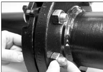
7. INSTALL REMAINING BOLTS/ NUTS: Insert a standard, full-shank diameter assembly bolt through each remaining hole in the flange adapter/ mating flange. Thread standard flange nuts finger-tight onto all bolts.
