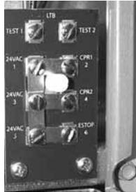
Voyager's Low Voltage Terminal Board is external to the electrical control cabinet. It is extremely easy to locate and attach the thermostat wire and test operation of all unit functions. This is another cost and time saving installation feature.
