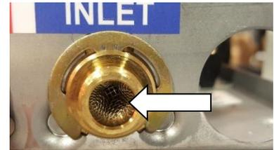
Remove the cover. Connect the pre-assembled inlet and outlet pipes to the heater (**do not overtighten compression fittings**) and fully open the inlet and outlet ball valves. Check the system for water leaks at all plumbing connections. If a leak is present at the compression fitting, **slowly** tighten compression nut until it stops – **do not overtighten**.
