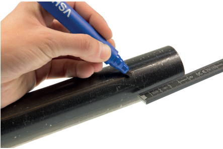
FIGURE 8: MARKING INSERTION DEPTH
