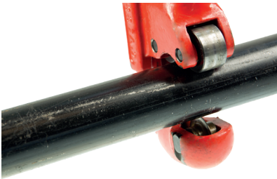
FIGURE 6: CUTTING THE PIPE
