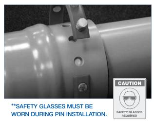
Using a 1 lb hammer, tap in the pins starting at the top of the pipe working your way down. The pins should be tapped until they bottom out on the inner groove or are flush with the ring. A good technique to ensure proper alignment is to tap each pin on the ring 1/4 to 1/2 of the way in before hammering in fully. If the pins will not go all the way in, check to see if the rings, holes, and inner groove are properly aligned on all sides.
