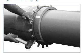
6 Check to make sure all of the pins are fully inserted before starting the next joint.
